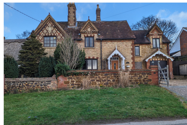
Coursed stone with brick posts, field gate.
